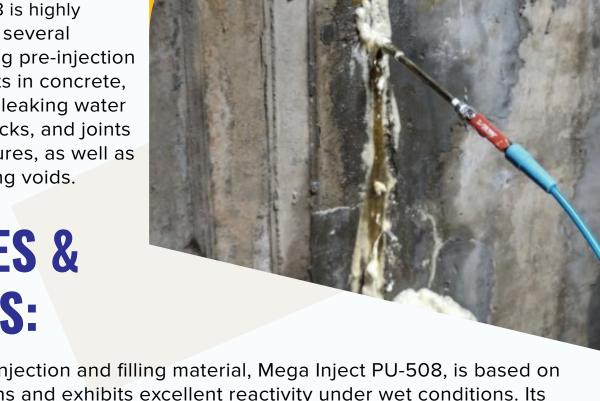
This solvent-free injection and filling material, Mega Inject PU-508, is based on Polyurethane resins and exhibits excellent reactivity under wet conditions. Its key features and benefits include reacting in moist surroundings, forming a strong bond with wet surfaces, and effectively stopping running water.
